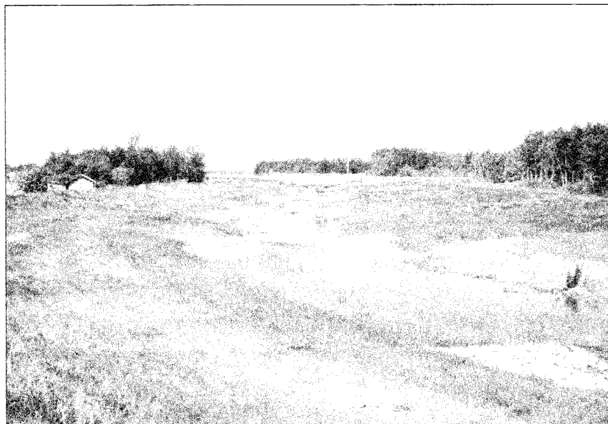
Figure 4-19: Stable spawning riffles and pools added to the rehabilitated reach of Mink Creek below Highway 20 under low-flow conditions in July 1988, two years after construction.
