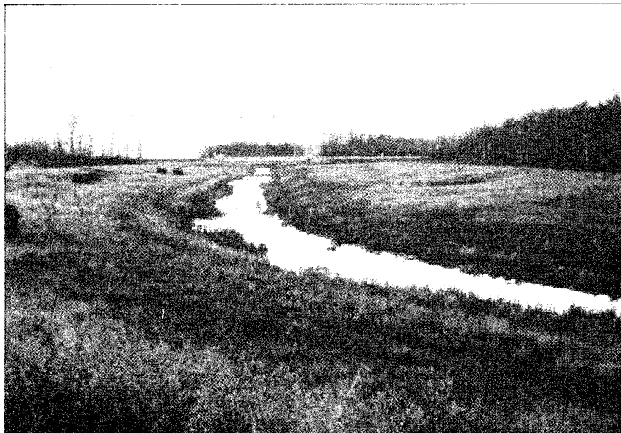
Figure 4-18: The uniformly channelized reach of Mink Creek below Highway 20 in September 1985, prior to the addition of spawning riffles and pools.
