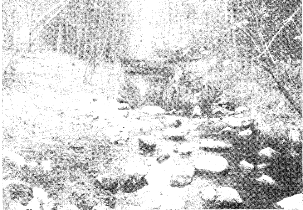
Figure 4-10: Upper spawning riffle and pool constructed in Hamilton Creek.
