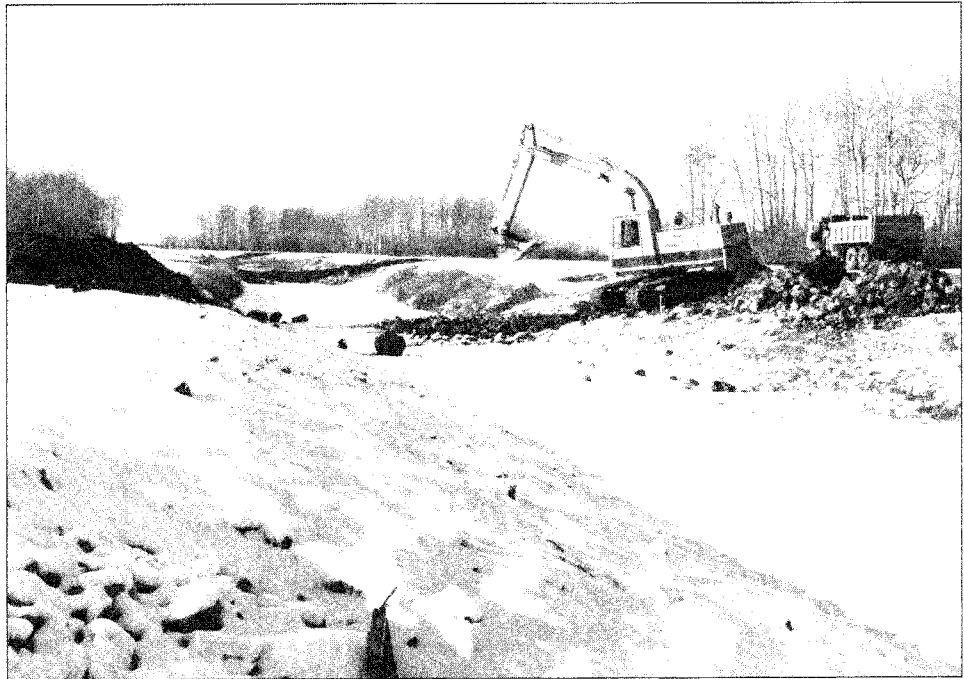
Figure 4-20: Mink Creek riffle construction above Highway 20 in November, 1985. A completed riffle is shown upstream.
